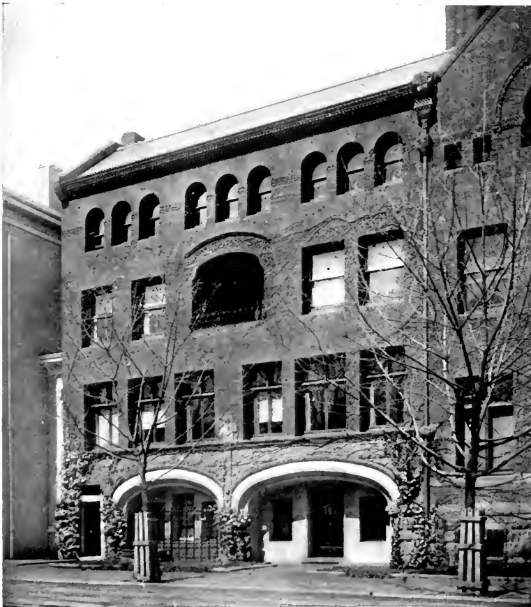
THE ADAMS RESIDENCE; PART OF A GROUP.
